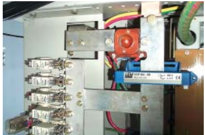
Fig. 8: HOP current transducer in a Chinese TeleCom application.
